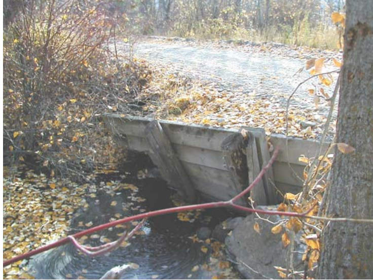
Figure 14. Failing culvert on Ronan Creek, 1999.
