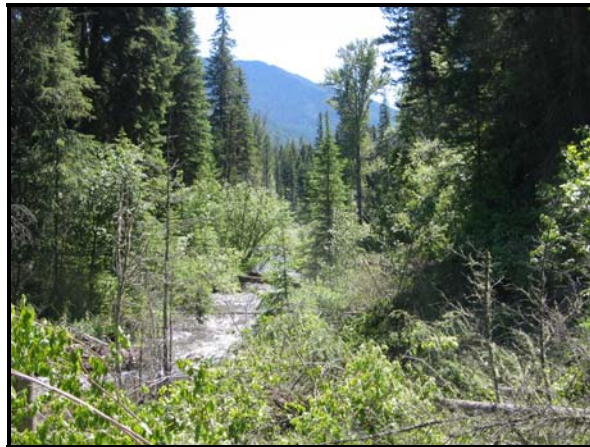
Figure 20. North Fork Jocko River following removal of the streamside road and transplanting of woody vegetation on the same site, 2004.
