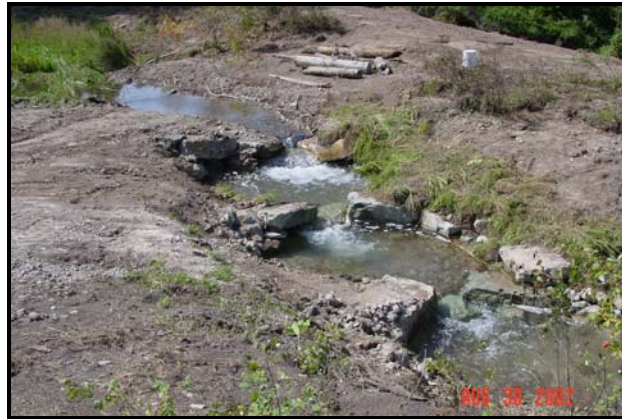
Figure 18. DuCharme Creek with in-channel steps through former dam site.
