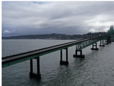
Deck Trusses and Girders
