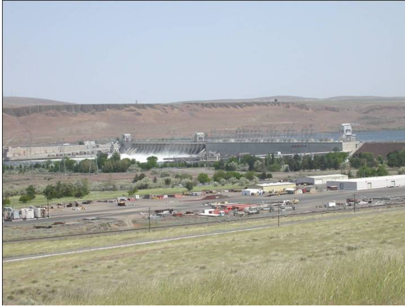
McNary Dam – spill, ladders, smolt by-pass, phase I ditch
