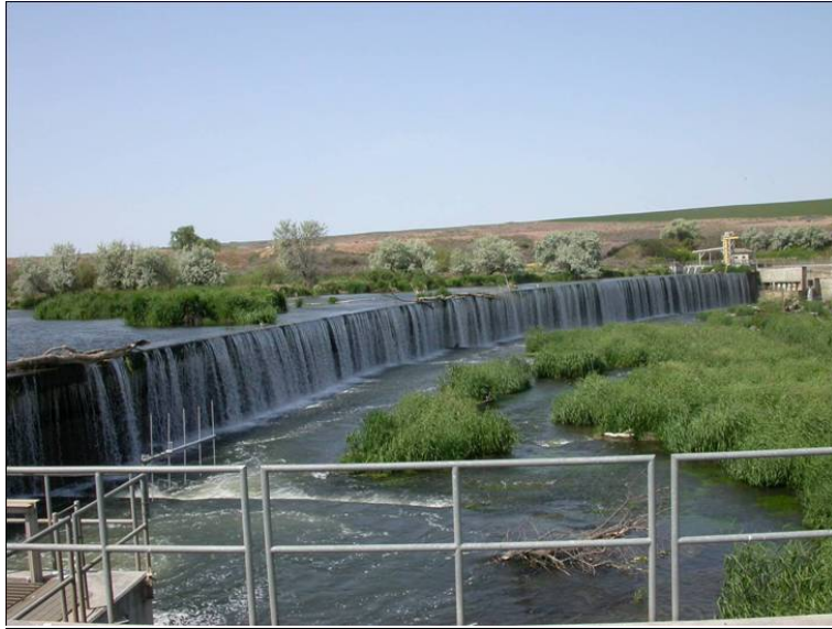
Three Mile Falls Dam
