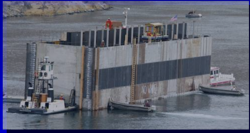
Rocky Reach Surface Collector being transported prior to installation
