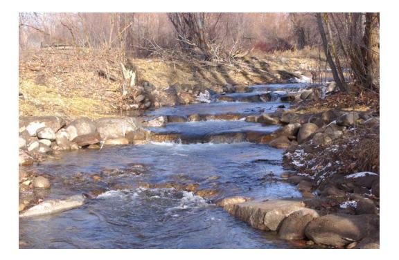
Figure B-6. Rock vortex weirs in Beaver Creek, Methow Subbasin
