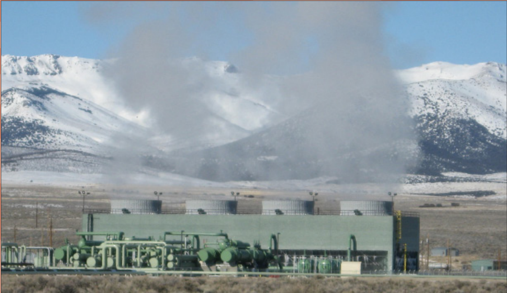
Raft River Geothermal Project
