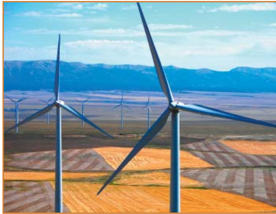
Judith Gap Wind Energy Center, Montana. Photo courtesy of NorthWestern Energy.
