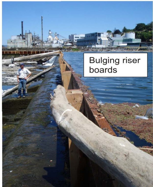
Figure 2. Installation of riser boards and lamprey ramps with HDX antenna at Willamette Falls, Willamette River, Oregon, 2010.
