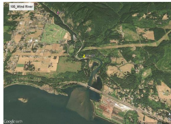
Address sediment build-up
