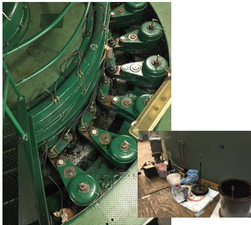
Wicket gates, in-line equipment, lubricated wires
