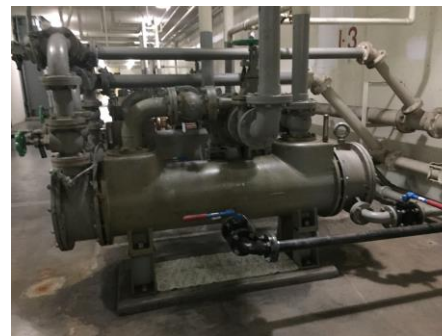
Cooling Water Intake Structures
