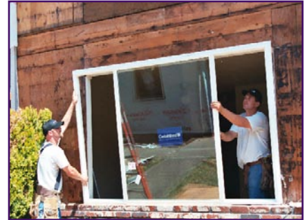
New energy efficient windows, installed by Richart Builders, will improve comfort and lower energy costs for tenants of the Rachel Anne Apartments. (Photo courtesy of Energy Trust of Oregon)
