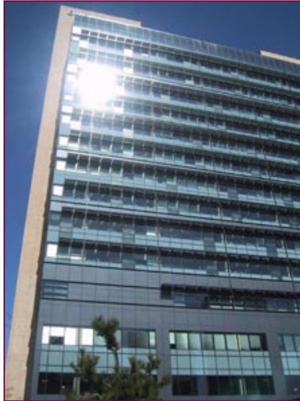
Oregon Health and Science University's Center for Health and Healing in Portland.
