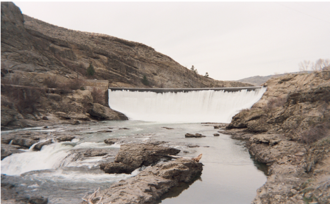
Figure 39. Enloe Dam on the Similkameen River.
