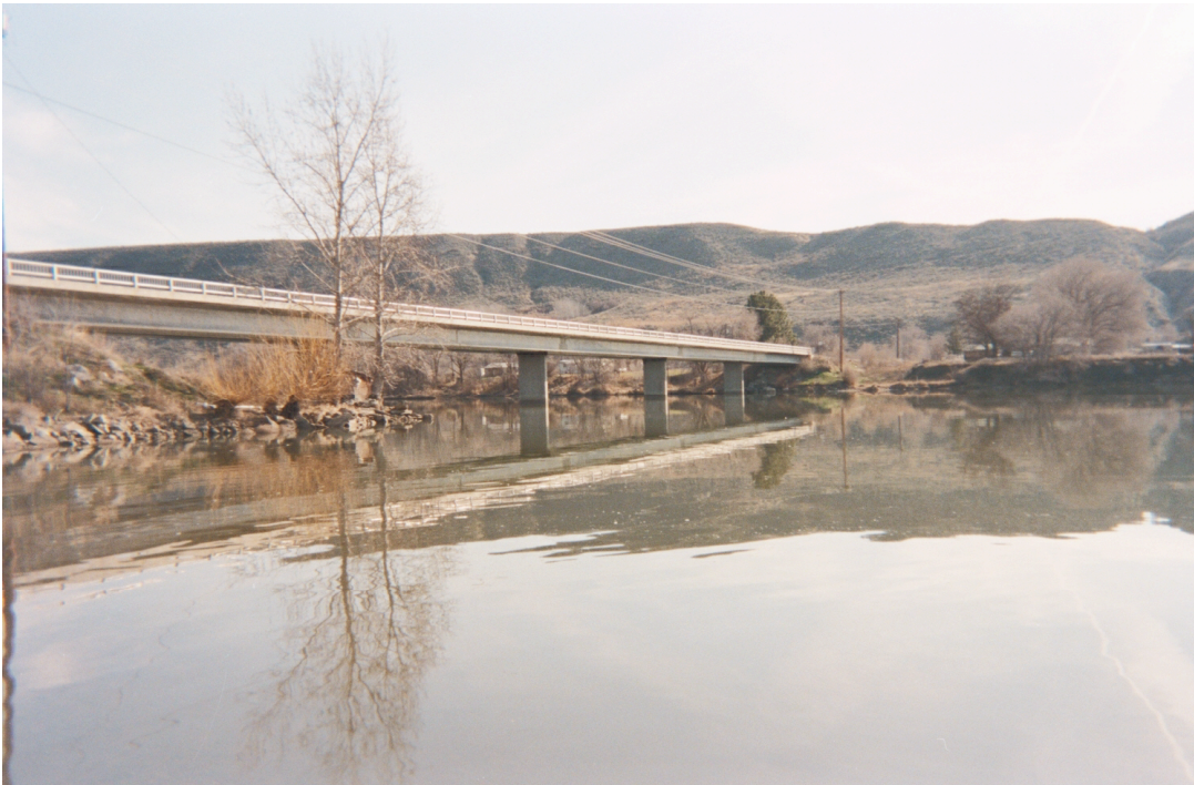
Figure 30. Monse Bridge on the Okanogan River, looking east.
