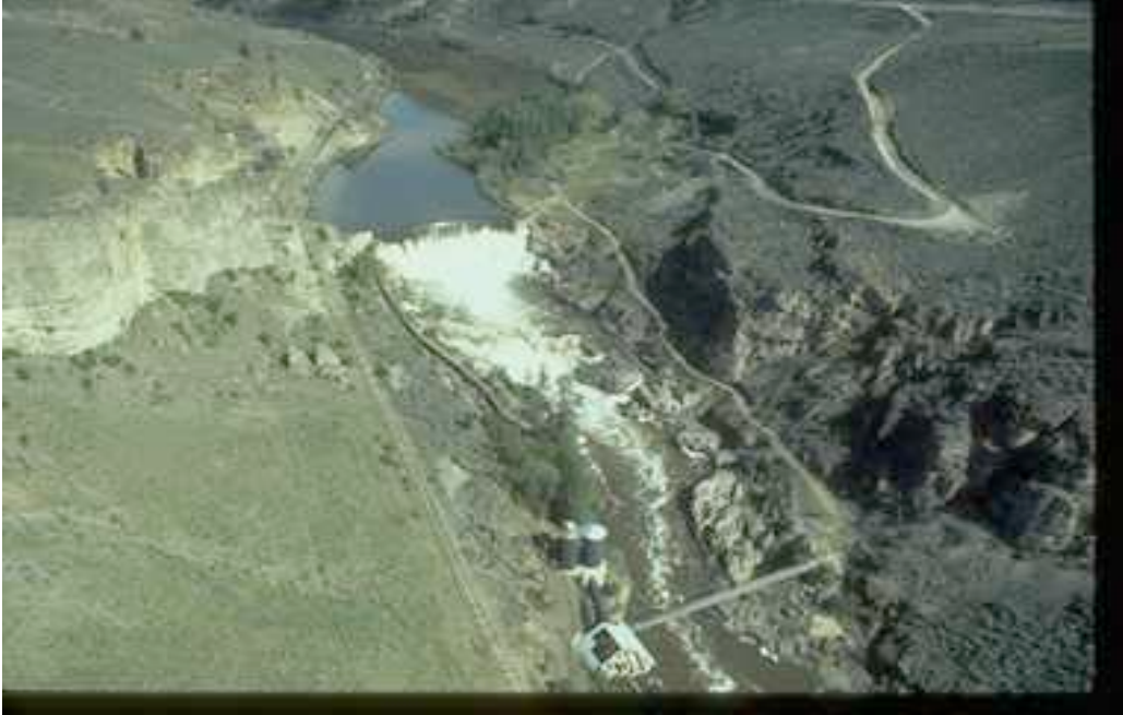
Figure 38. Overview of Enloe Dam (streamnet.org).
