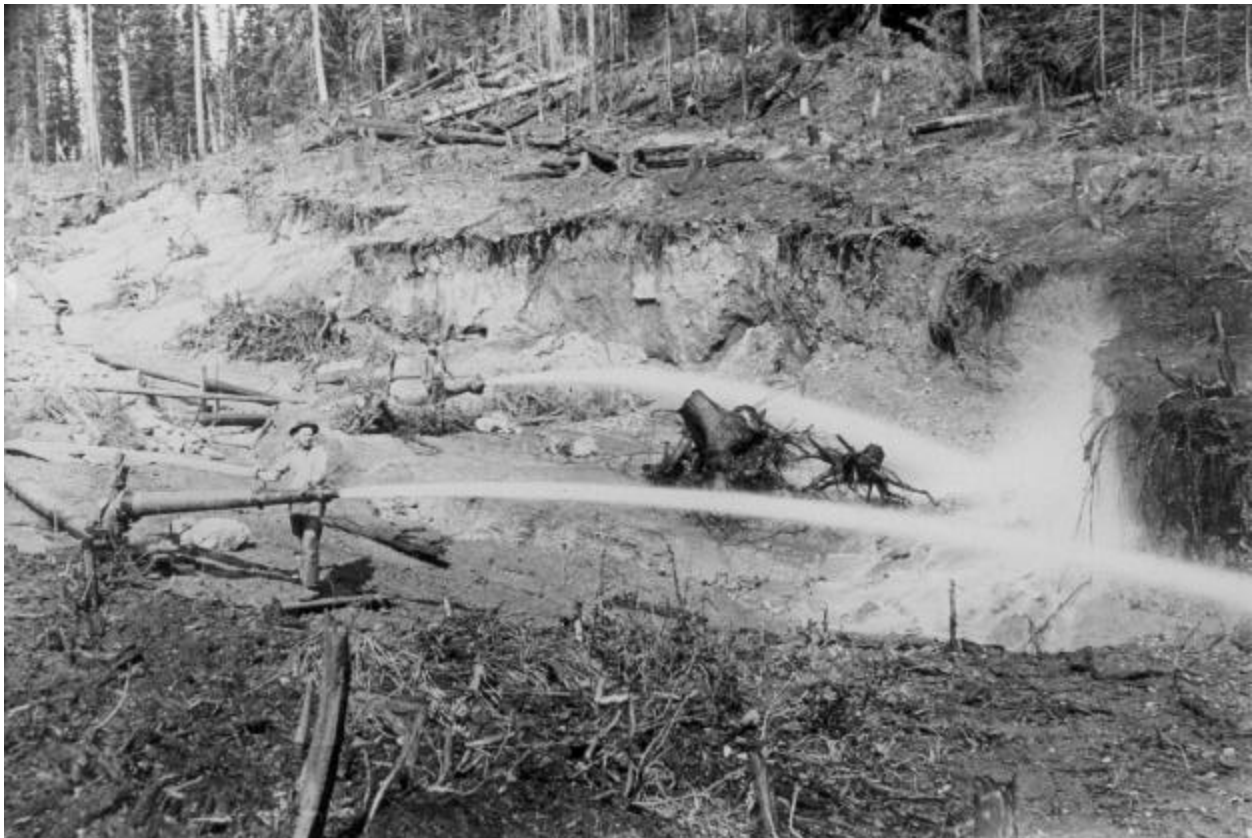
Figure 39 Hydrologic mining on Leggett Creek in the South Fork Clearwater drainage (photo courtesy of Don Morrow)
