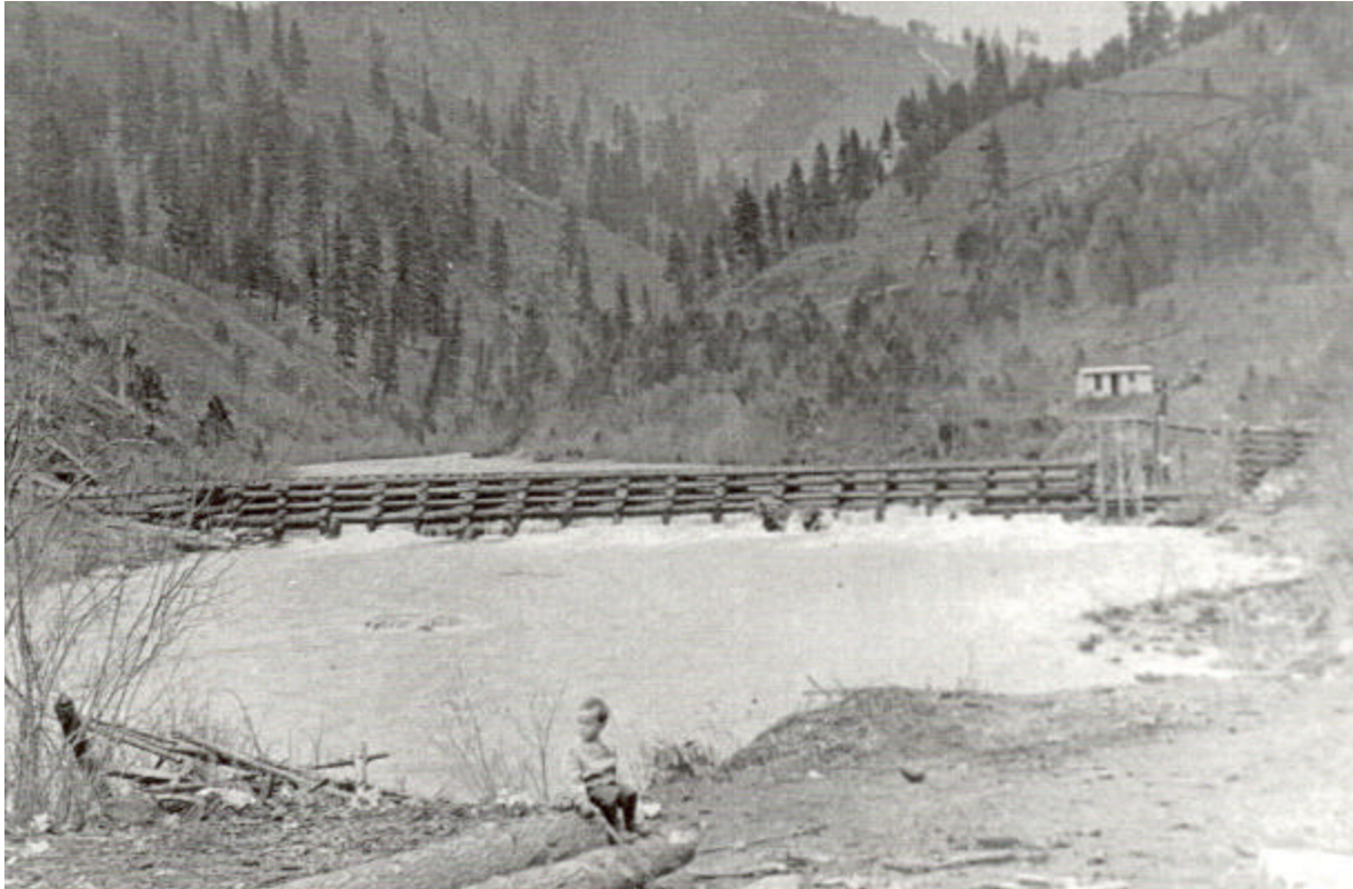
Figure 43 Dewey Dam (Courtesy Don Morrow)
